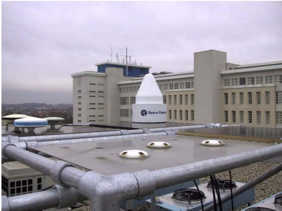
**Figure 3. Space Engineering antenna mounted on the rooftop of the Septentrio office in Leuven.**
